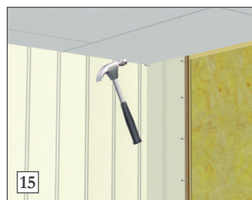
15) The panel is nailed in the nail lip. In the corner, the panel is nailed visibly with dive pins (by hand). Secure top and bottom as usual. Use correction paint (in correct colour) to cover the visible nails.
